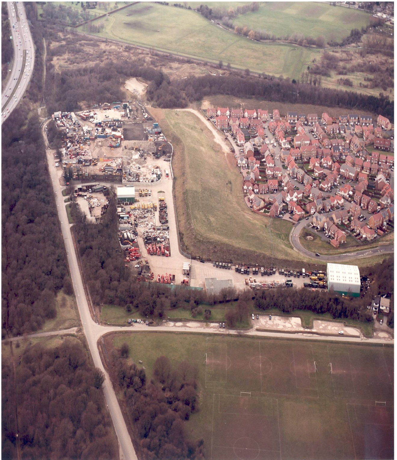
Figure 3 - Aerial photo showing the site in its wider setting
